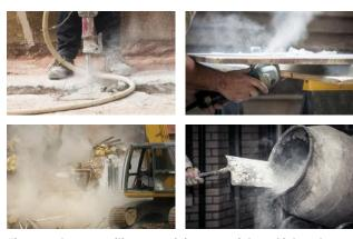
Figure 1: Common silica-containing materials and job tasks where you may be exposed to silica dust
